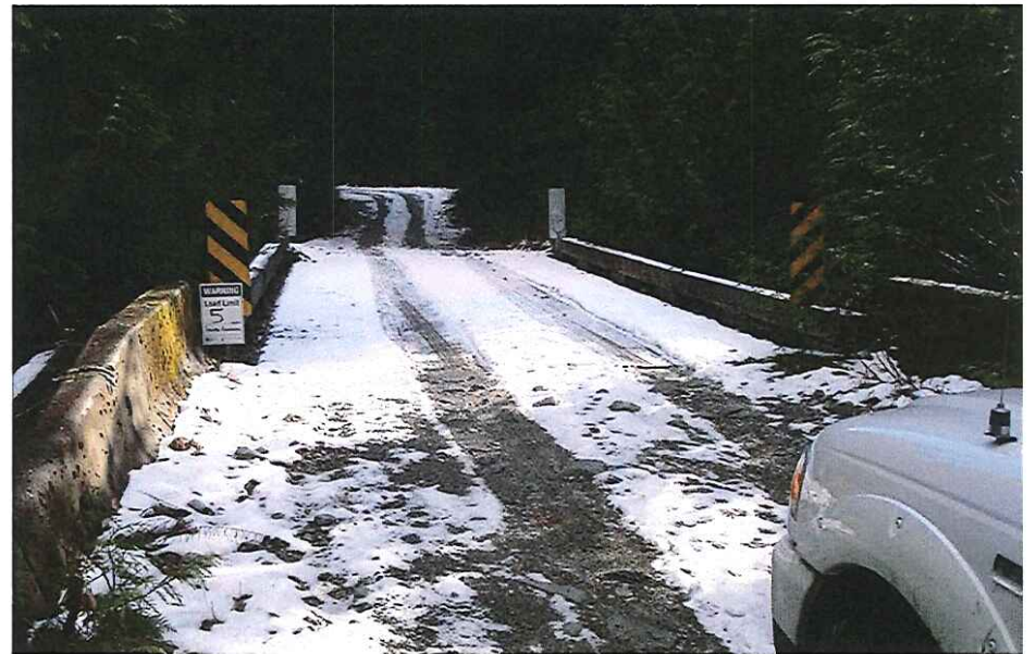
CK2178 Approach Right Bank
