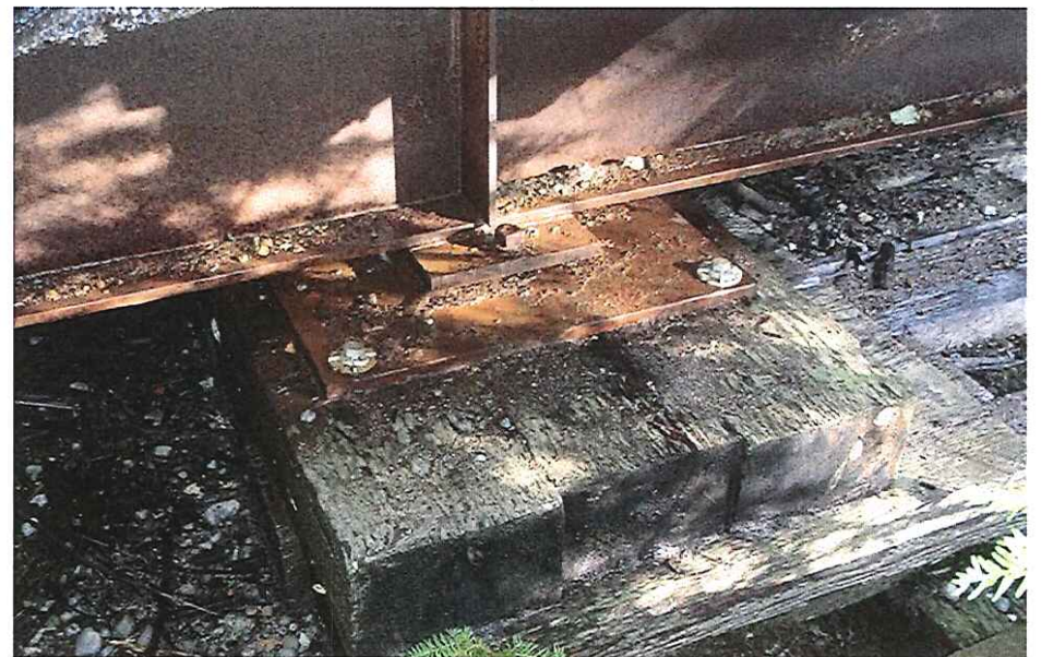
CK2178 Bearing right bank to portable bridge
