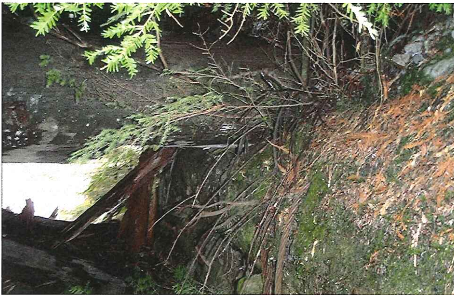
CK2178 Abutment Left Bank
