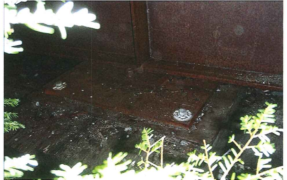
CK2178 Abutment left bank to portable bridge
